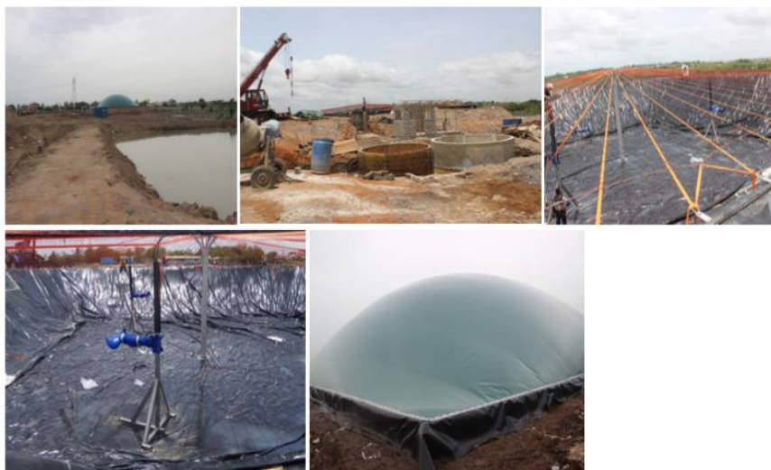
Figure 8: Stages of construction of Waste to energy plant in Ashaiman
